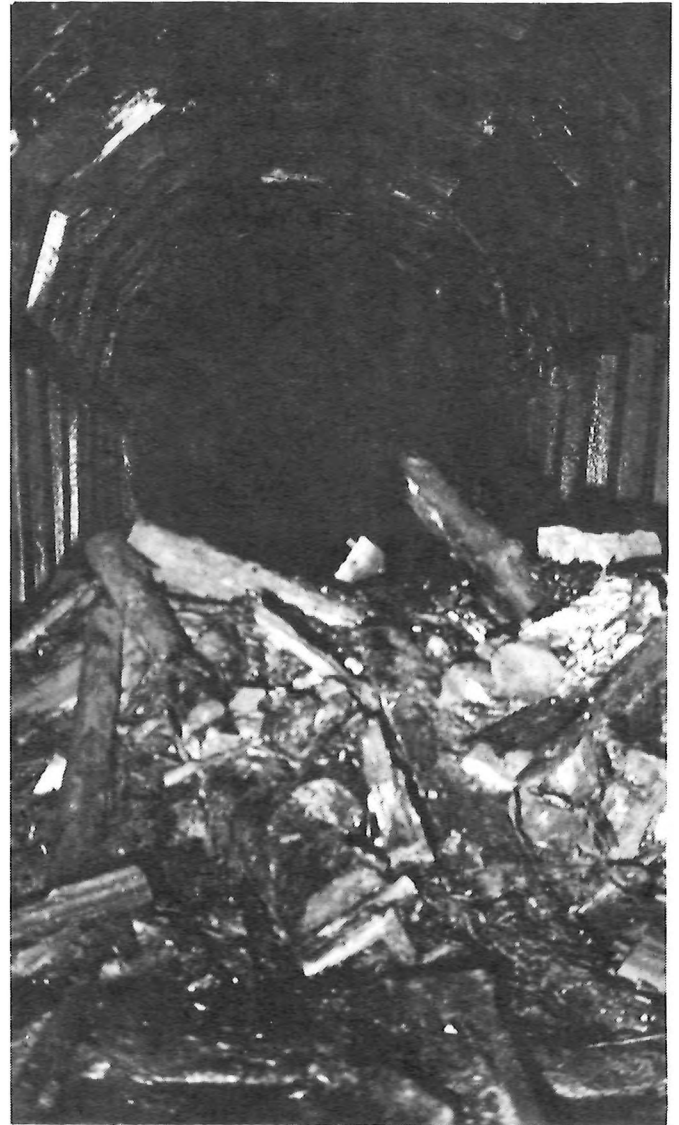
A rockfall inside the Alpine Tunnel that was encountered during the October 2, 1948 visit. (Ed Haley Photograph)
