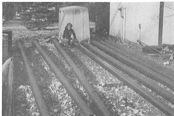
Rail joints on electrified track must be double wire bonded to insure a good ground circuit. Here Club member Dave Waltrip performs one of the many welding jobs that were necessary. (DTA)
