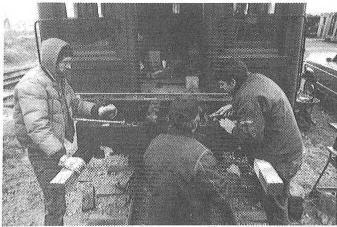
Although members of our organization were able to donate time to the Ft. Collins project during this fall, the Club's equipment was not being ignored either. Here we see Tom Caldwell, Bill Gould and Dave Waltrip busy reassembling the completely rebuilt rear platform on the Club's narrow gauge business car RICO. (Your equipment donations at work!!!) (Darrell Arndt Photograph)
