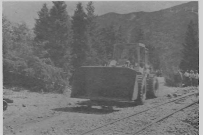
"To the rescue" This frontend loader was finally brought in to help lift the car back onto the rails using chain.
