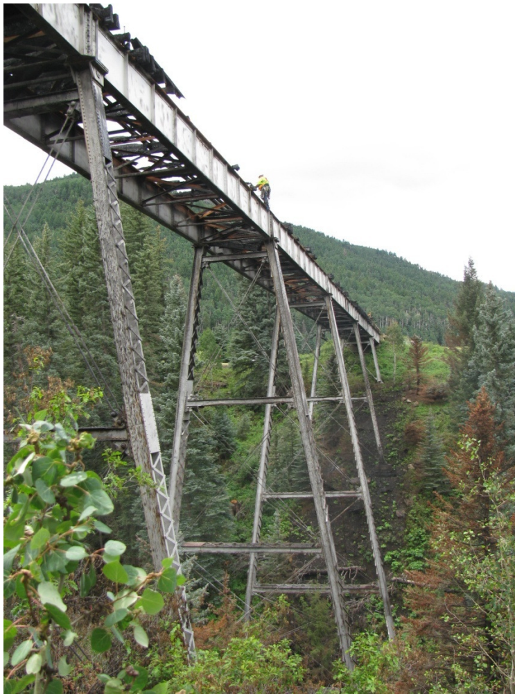
North face (left Side) of bridge Looking Timetable West toward Chama
