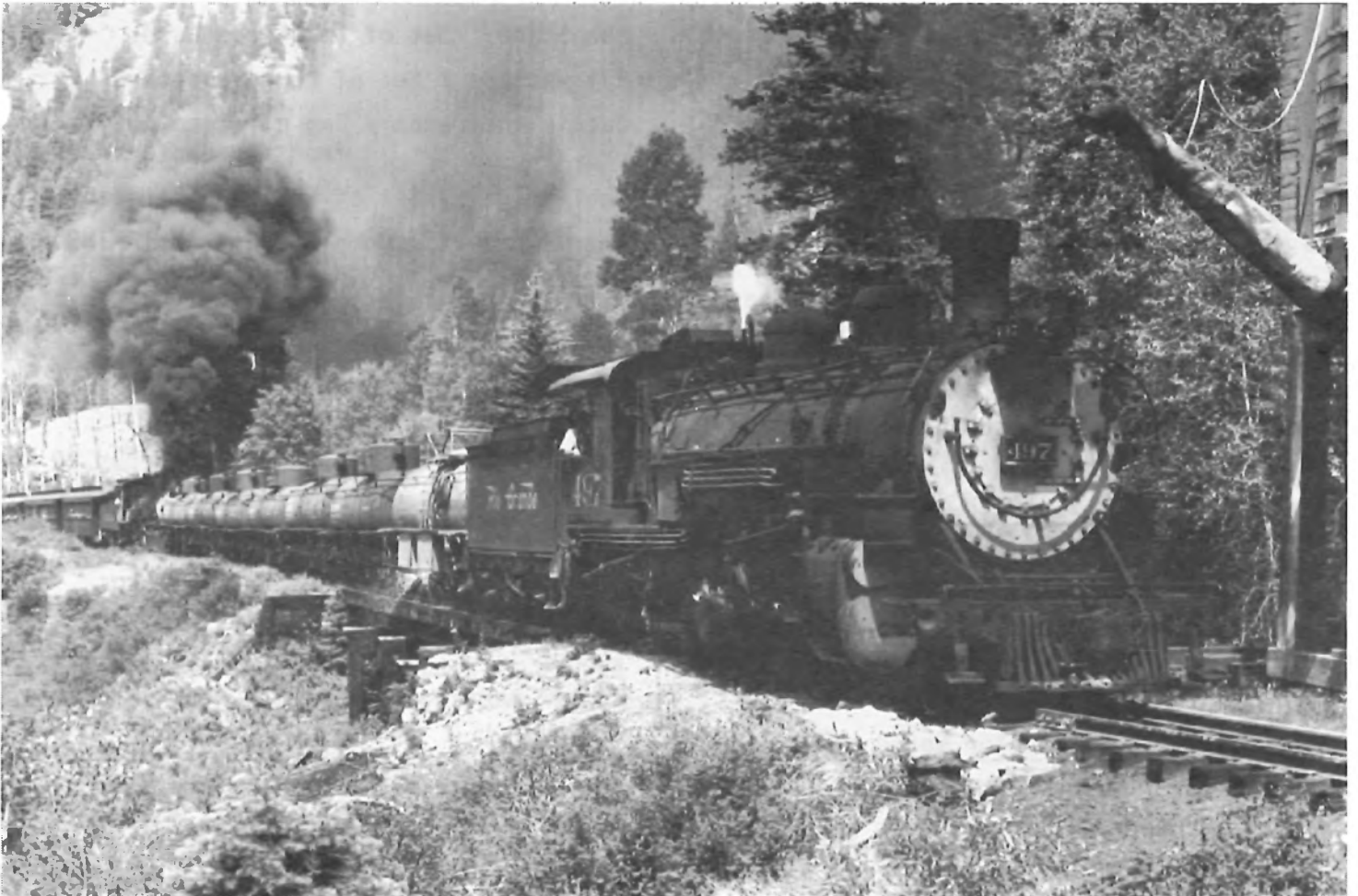
June 29, 1996, saw engines #497 and #489 pulling the regular train and some freight cars up to Cumbres. The tank cars were part of a special freight train run by John West on Sunday, June 30, 1996. Cars had been set out at Cumbres during the week to create a 22-car train on Sunday's Big Horn Wye Turn with several engines being used throughout the day. Note water car #0472 in the consist. It has been used in fire control service, spaying water out about four feet on each side of the train to reduce spot fires. The location is Cresco Water Tank. (Jim Trowbridge Photograph)
