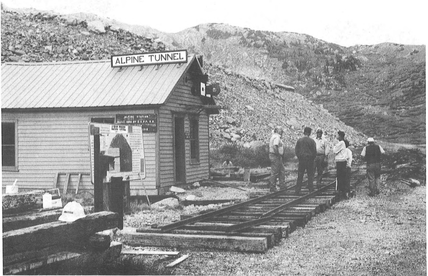
Rail once again rests on the roadbed of the famous Denver, South Park & Pacific Railroad as a stretch of track is laid in front of the Alpine Tunnel Station at the west portal of the Alpine Tunnel on August 19-20, 1994. (Ron Keiser Photograph)
