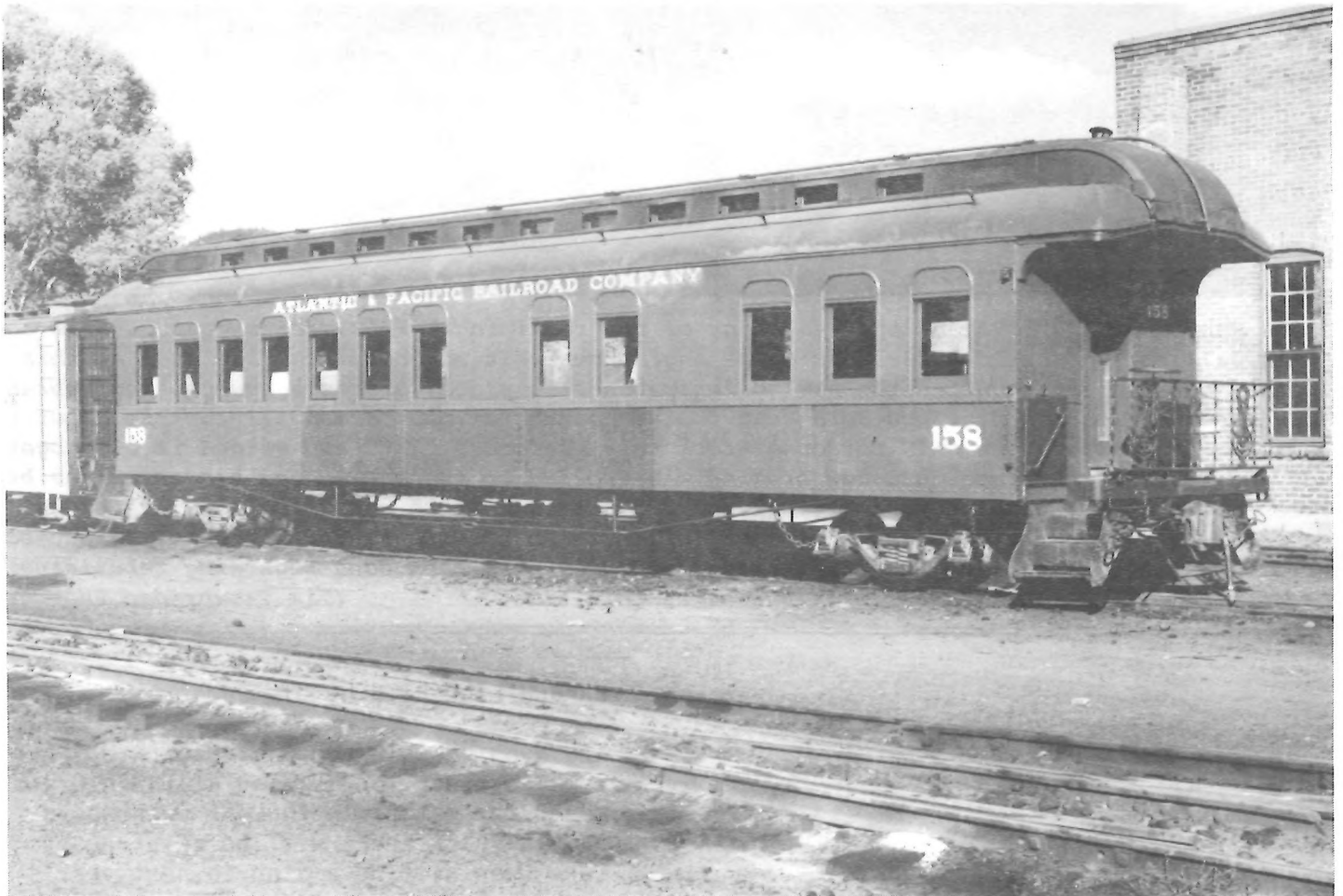
The "Hinman" car, an ex-Mexican narrow gauge passenger car was extensively repaired, restored and repainted for Kevin Costner's new movie, Wyatt Eary . Besides the interior work, the exterior received new "siding" to resemble the look of a steel-sided car (leave it to Hollywood to want an 1880's passenger car to have steel siding rather than the actual passenger-car wood siding!). Sheets of Masonite (R) were applied with rivets to simulate the steel siding. The coach looks beautiful! (Jim Trowbridge Photograph)
