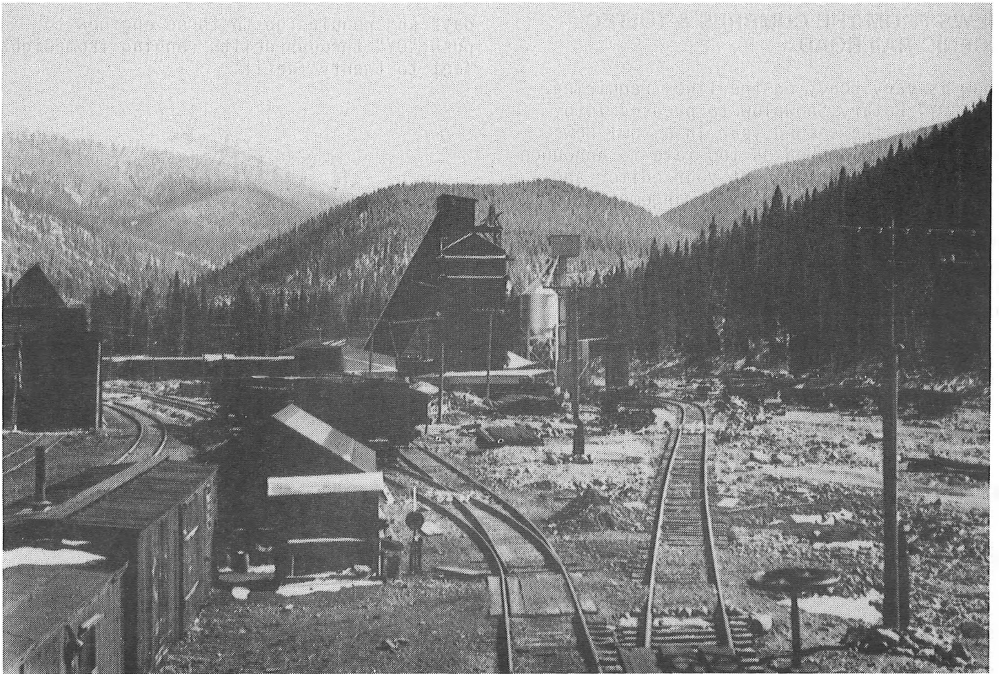
Concrete Plant, West Portal of the Moffat Tunnel
