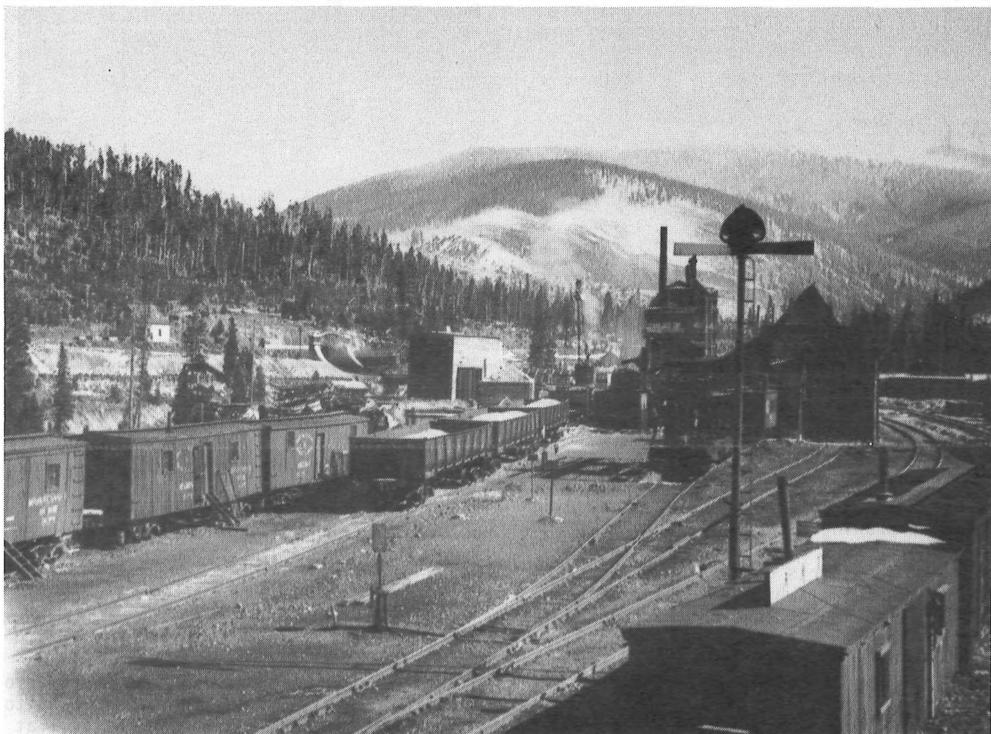
Two scenes of the activity at West Portal (Moffat Tunnel) in September, 1935, showing the M-O-W car West Portal Station with the semaphore and the concrete mixing plant. During 1935, the Denver & Salt Lake almost completed the concrete lining of the Moffat Tunnel; at the end of the year, only 250 feet of the lining remained to be completed. While this was underway, the Denver Water Department was working to complete lining of the Moffat Water Tunnel, seventy-five feet south of the railroad tunnel; this project was completed nine months later. [Research and writing of the Moffat Tunnel history progresses with plenty of material to complete the story--Bob Griswald] (Denver Water Department Photographs)
