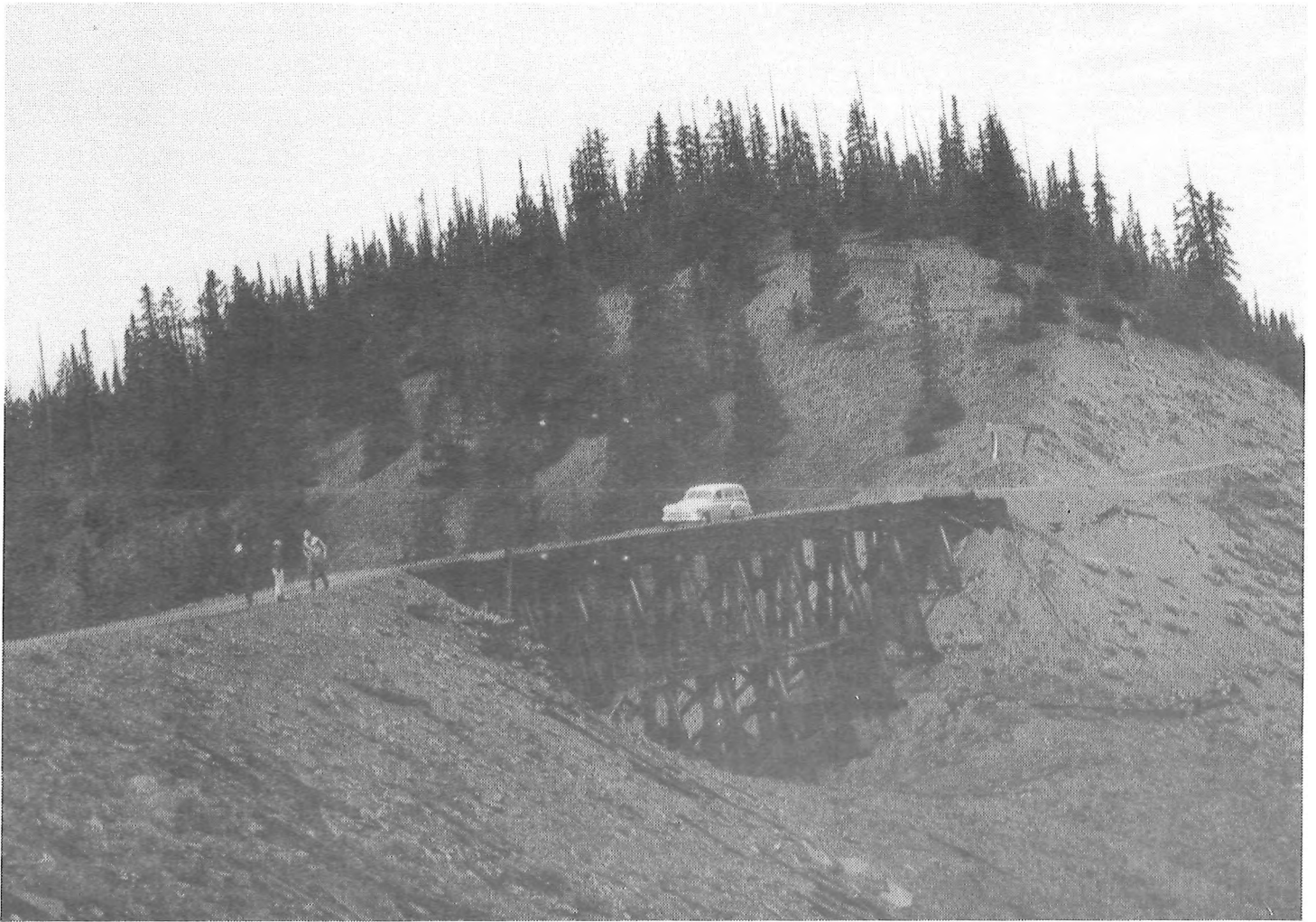
At Riflesight Notch, the railroad crossed over itself by means of a trestle built right over a tunnel just beneath. Clarence, our driver, gingerly eased the station wagon across while some of us chose to walk. August 10, 1952. (Irv August Photograph)
