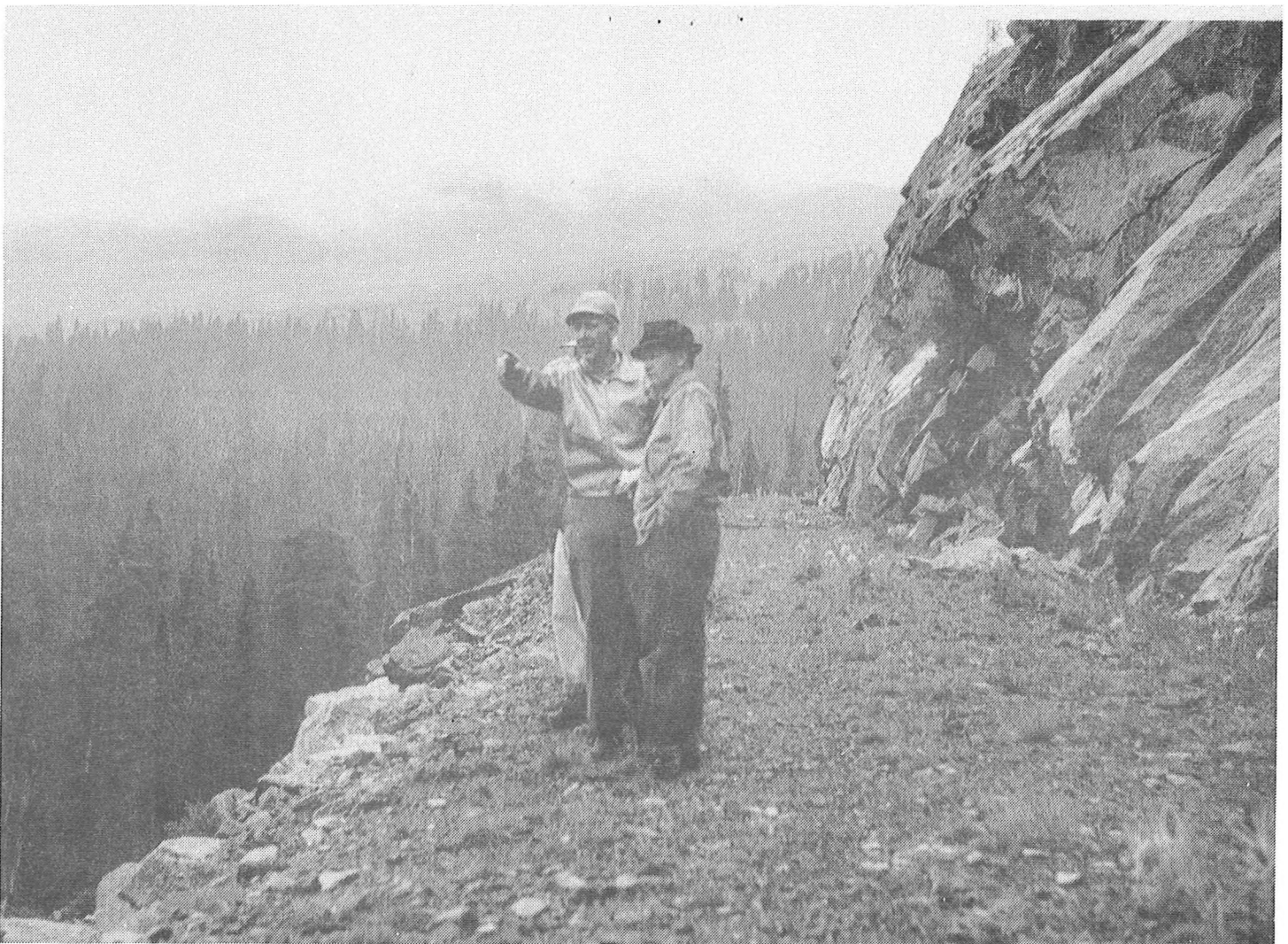
Danny Peterson points out the site of the wreck of number 210 to Les Logue. It was here, just below Riflesight Trestle, on the shelf railroad grade that the 210 left the rails in December, 1924, and plunged hundreds of feet to the canyon floor. It was later recovered by means of a 30-degree "Shoo-fly." (Irv August Photograph)
