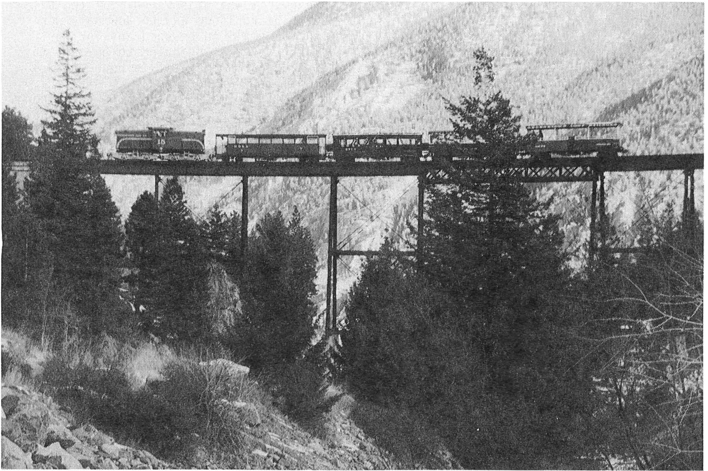
Georgetown Loop Railroad Diesel No. 15 is shown bringing its train over the Devil's Gate Bridge (trestle) on the first run, December 7, 1991. Several RMRRC members were on hand to ride the train. (Sherm Conners Photograph)
