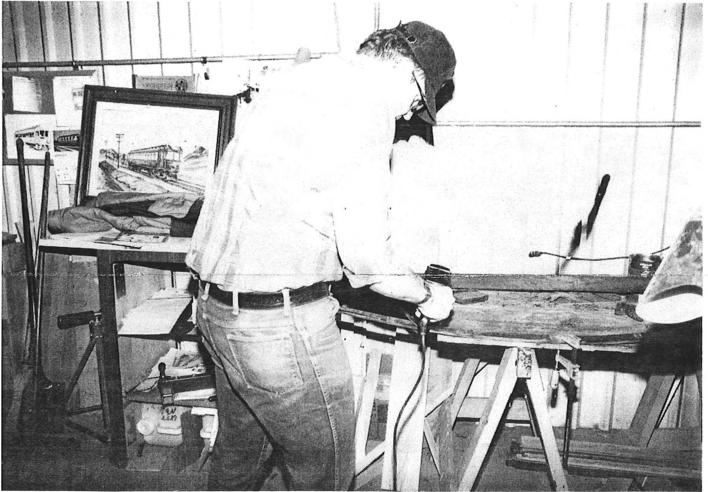
Joe Priselac is hard at work stripping old paint and varnish from clerestory roof end slats in hopes of preserving as many as possible, although many will have to be replaced with new material, requiring "steam" shaping. Note the painting just to the left of Joe. Joe is quite an accomplished artist and has painted the No. 25 as it would have appeared in its early years and how the Club hopes to have it appear in the very near future. Perhaps we can have Joe bring his painting to a future meeting for everyone to enjoy and provide an insight into how the No. 25 will appear in the future!! [Jim Trowbridge Photograph]
