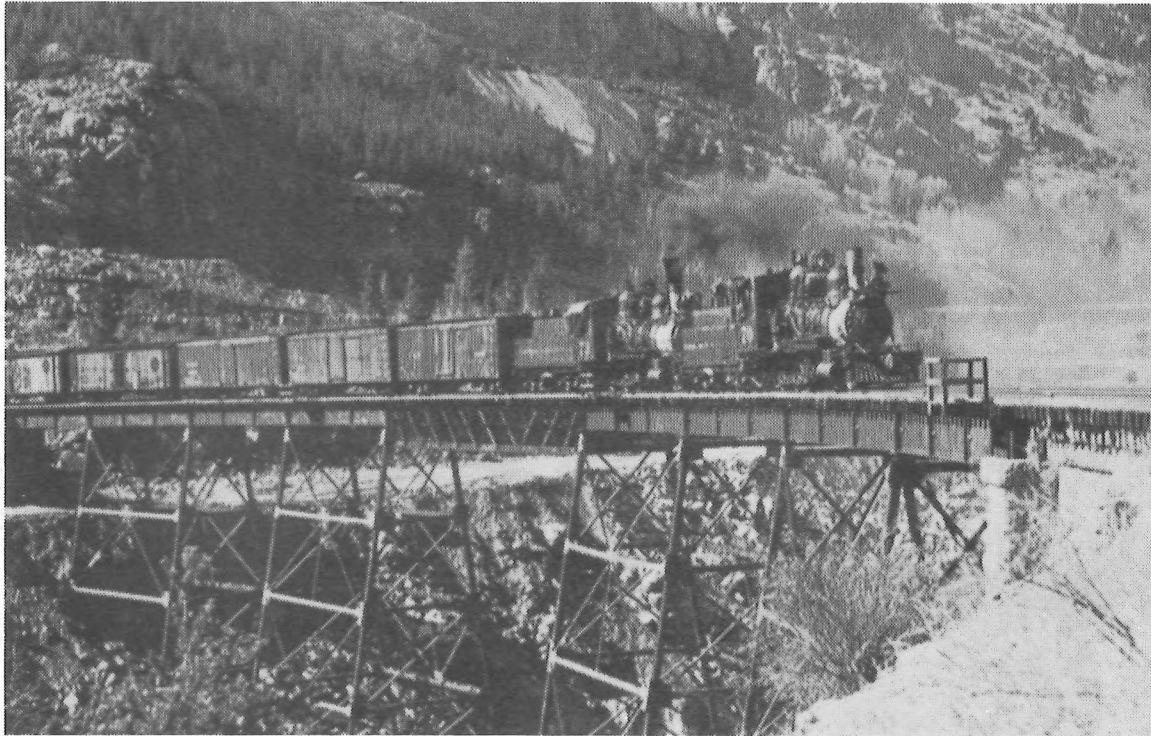
Colorado and Southern engines 70 and 73 doublehead a westbound freight over the high bridge on May 14, 1938. Less than a year later, the last train would cross the bridge. A comparison of this photograph with older pictures of the bridge will show how the structure was strengthened in the early 1920s.
