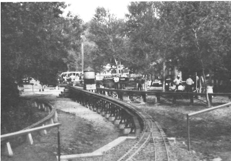
Here we see the completed Wye. The trackwork in this area is something to behold. Dual gauge (note the switch entering the trestle and the track on the trestle), crossovers, switches, yard tracks--it was a modelers delight! The Pole Barn, center right, is the new Jerry Cutshall Hall. (Jim Trowbridge Photograph)
