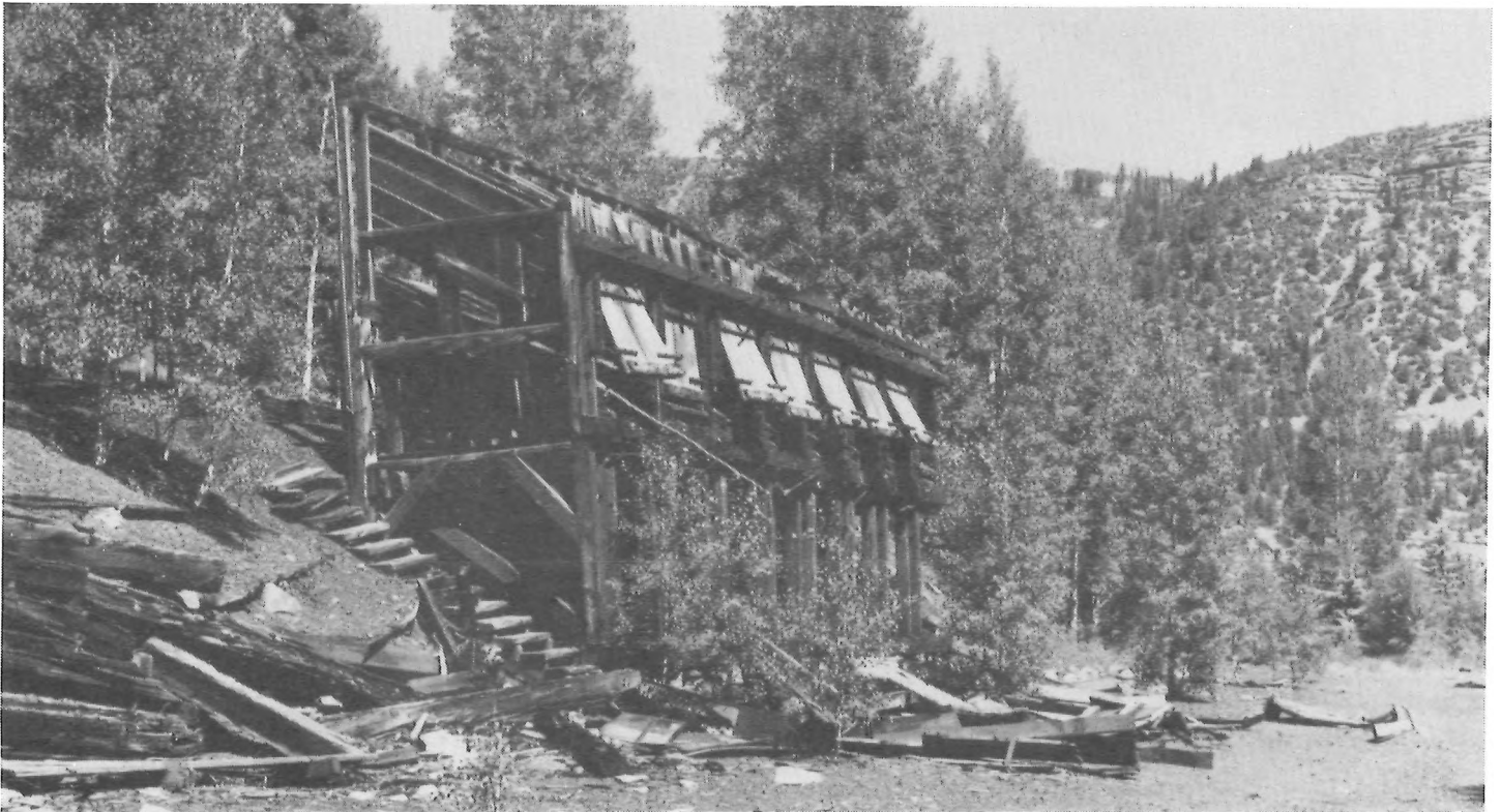
The Coaling Dock and Pockets at Vance Junction. This is a fascinating structure and there is enough left to explain the full operation of coal loading from the upper, back level into the storage pockets for eventual engine use. A coal storage dock is also located on the upper back level. (Jim Trowbridge Photograph)
