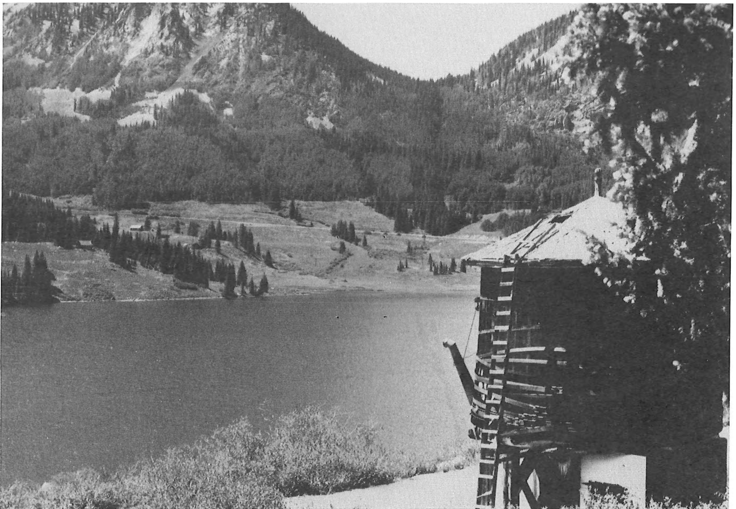
A spectacular view of the Trout Lake Water Tank on the Rio Grande Southern, looking out across Trout Lake. The RGS roadbed is, of course, just in front of us and one can travel on it for several miles in either direction from this point. (Jim Trowbridge Photograph)
