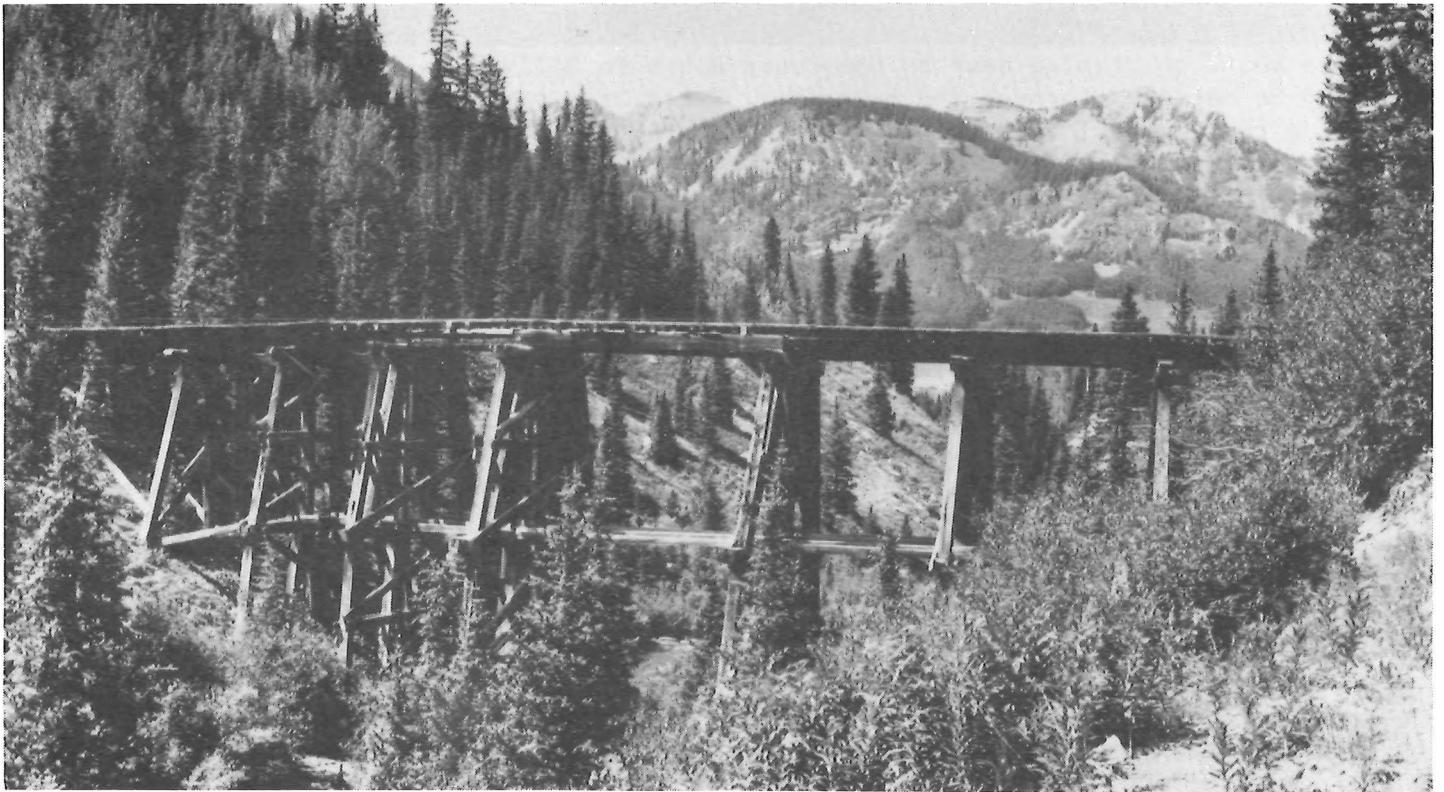
While a few trestles still remain in tact along the RGS right-of-way, this one is the most spectacular and is located about a mile or so above the Trout Lake Water Tank, on the way to Lizard Head. (Jim Trowbridge Photograph)
