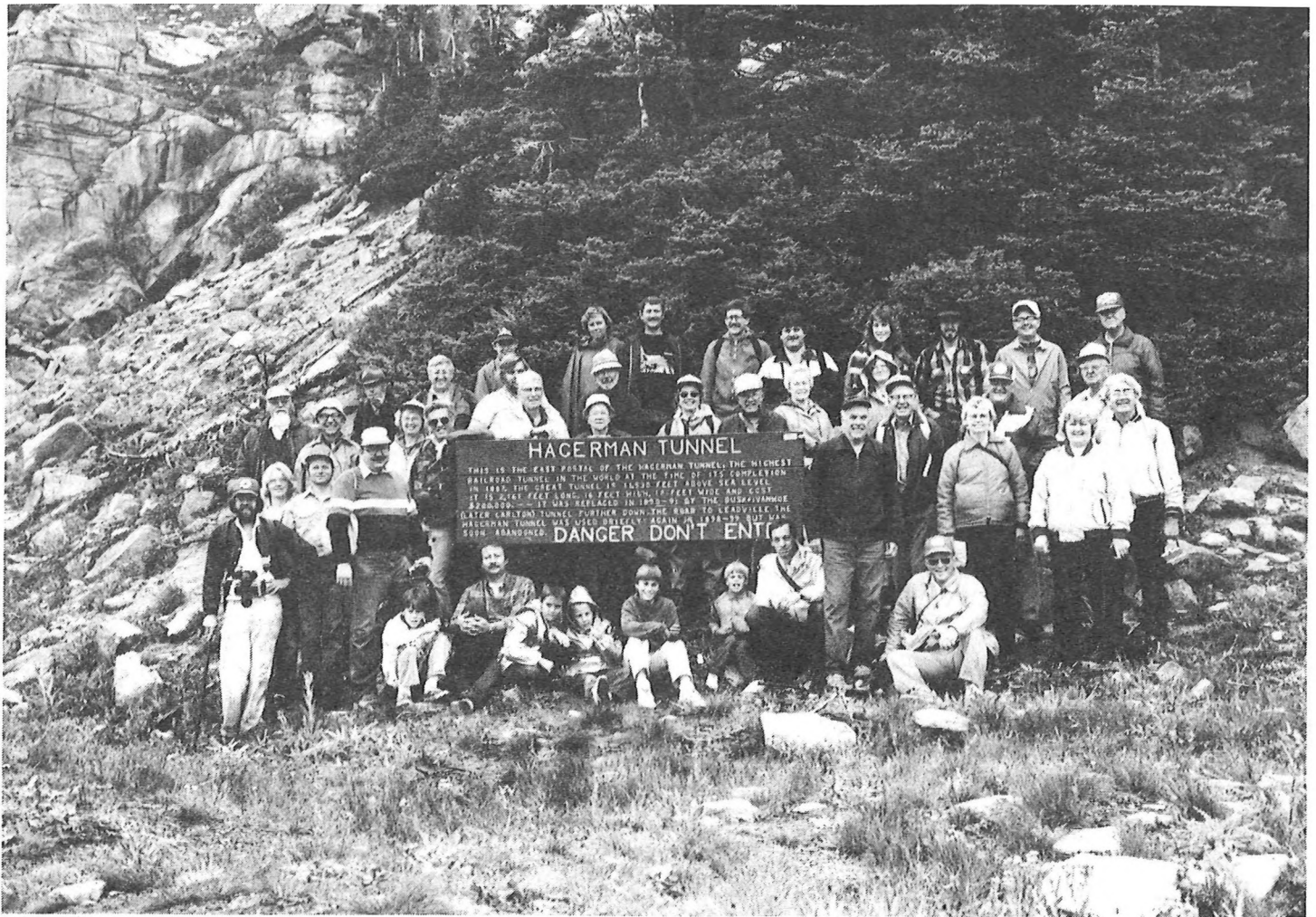
A hearty group lines up for a photograph at the East Portal of Hagerman Tunnel on the Club's August field trip over the roadbed of the Colorado Midland Ry. on the eastern slope of Hagerman Pass. (Tom Lawry Photograph)
