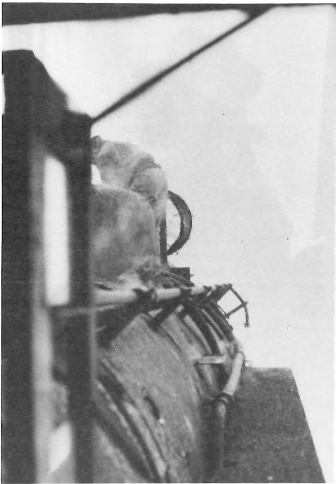
Being an engineer isn't all glory. Here we see Earl having to lean over the smoking stack, trying to replace the spark-arrester. It turned out that some brackets had broken and Earl had to leave it off. No matter today! Will this snow storm, the fire danger is virtually non-existent. (Jim Trowbridge Photo)
