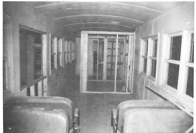
This is a view of the former coach, Capulin , which is being refitted into a coach-restroom-handicapped car. You are looking at the new restrooms, one regular, and one for the handicapped being framed in while a side opening is being created for a lift for the handicapped. (Photo by Jim Trowbridge)
