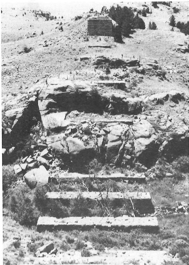
From the east abutment of the Dale Creek Bridge, one can easily put the abutments and massive pier foundations into perspective. (Darrell T. Arndt Photograph)
