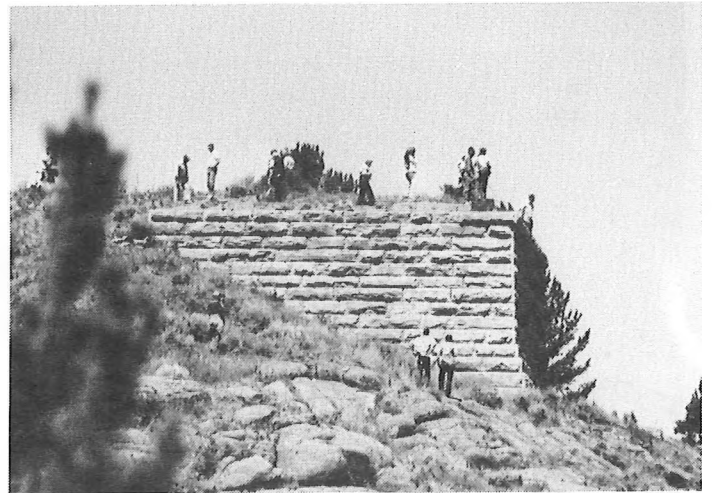
The west abutment is quite impressive and in remarkable good shape after all these years. (Darrell T. Arndt Photo)
