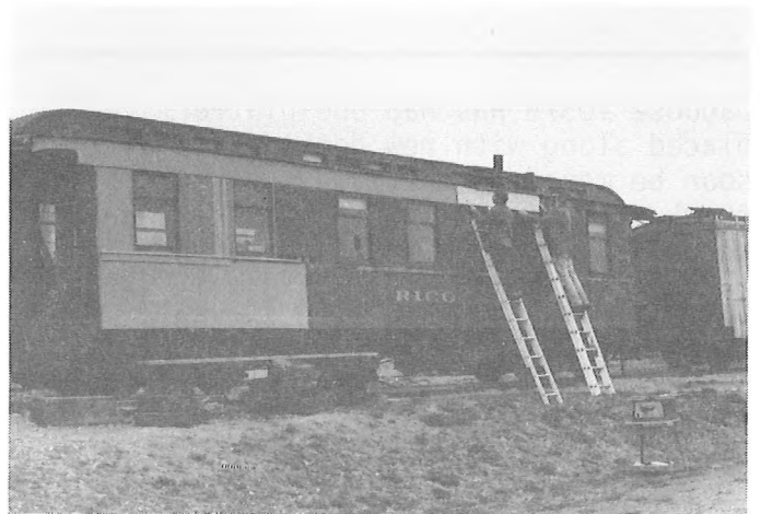
Bill Gould and Dave Waltrip fit a new piece of letterboard on RICO. Note the new siding, belt rail and clerestory siding. Rich Berens was also out this day and was helping Bill and Dave on RICO.
