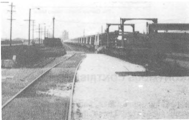
Rail train receives welded rail. Because lead-out strands are adjustable both horizontally and vertically, the strings can be fed into any one of 40 pockets on the rail train, which has roller racks for 10 rails across and 4 rails high. Second track to left of train in photo will permit loading two trains alternately without immediate switching.
