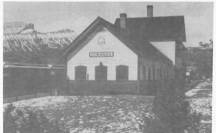
The Durango Station in the relative quiet of late fall. The winter train has already left for one of the few remaining trips all the way to Silverton and back.
