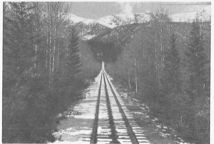
One of the very few straight stretches on the line, we can see a good grade ahead.
