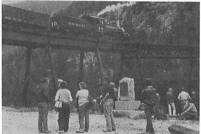
The old commemorative marker still stands and marks a good spot to view our train about to run out onto the high bridge again.
