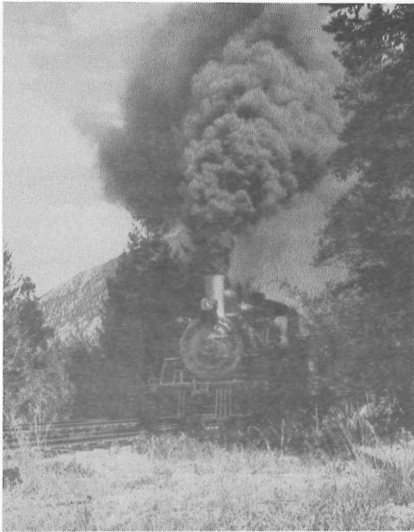
Our first photo run-by was held in the area of the Hall Tunnel. The engine crew gave us quite a fine runby with plenty of whistle, smoke and the music of a hard-working steam locomotive.
