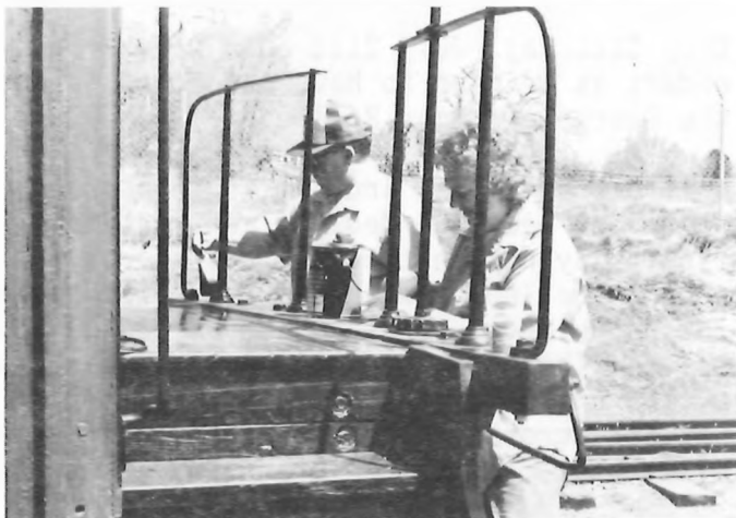
Cyndi Trombly and Jack Morison made sure that the RICO got a new coat of paint on the new end platform. Electricians are fine, but Jack likes the narrow gauge.
