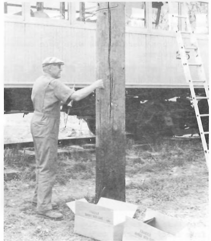
Carl Carlson works at a feverish pace. He ran out of equipment to caulk, so this trolley pole looked like it could use his attention. (Actually, Carl was trying to get the dried caulking off his fingers)
