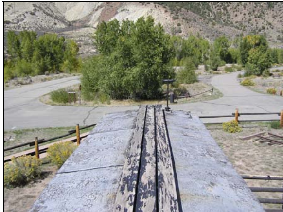
Figure 114. Roofwalk looking A end to B end
