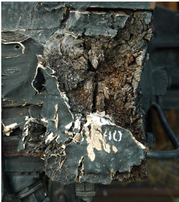
Figure 108. Right side A end rotten end beam
