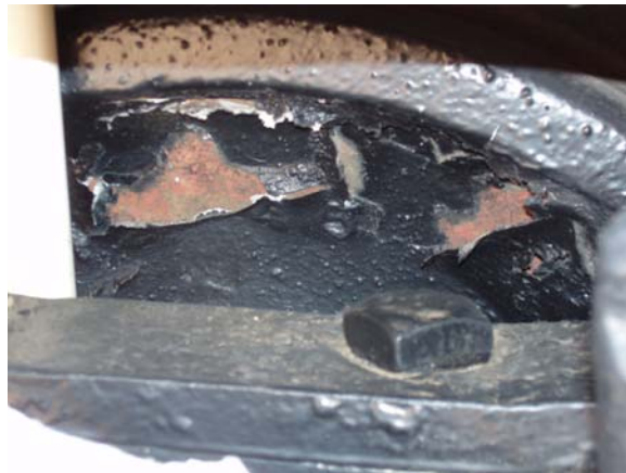
Figure 81. Rust and paint peeling on wheels
