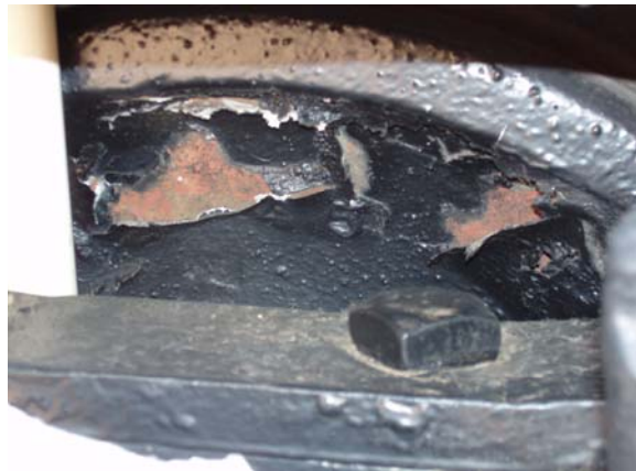
Figure 65. Peeling paint and rust materials
