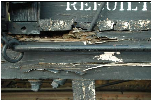
Figure 107. Right side B end rotten cross bar
