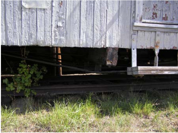
Figure 124. Rotten wooden beam
