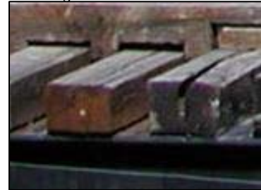
Figure 30: Weathered ties
