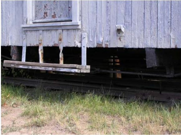
Figure 123. Deteriorated foot board on the side
