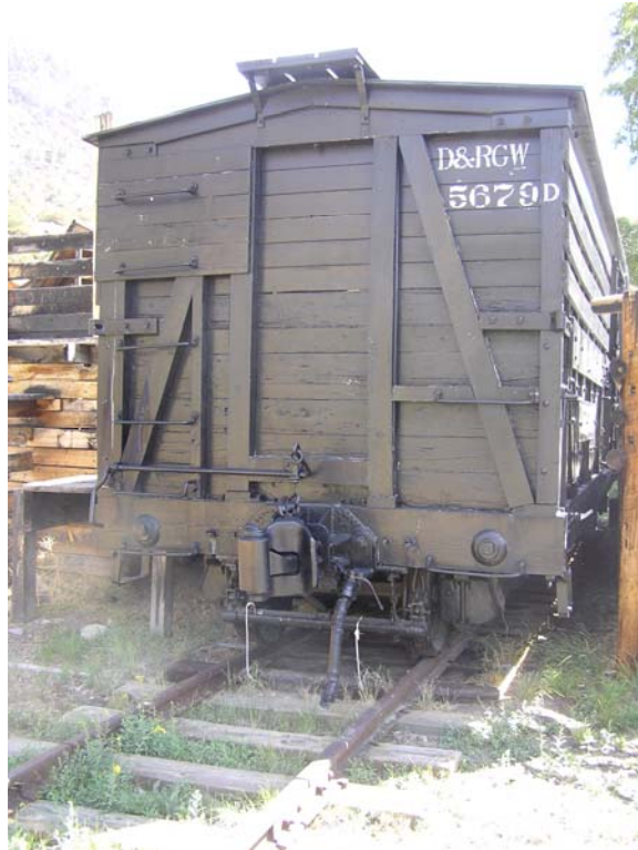
Figure 115. View of A end, Conditions of A, B end are good comparing to the other cars
