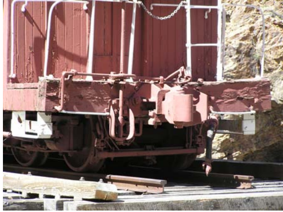
Figure 102. Bent B end's sill
