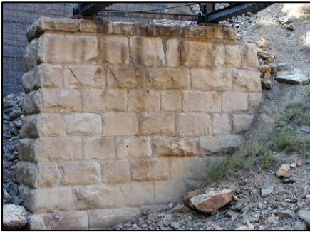
Figure 29: Missing capstone
