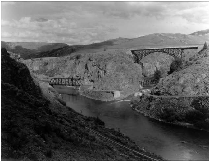
Figure 5: Bridges at Lake Fork
