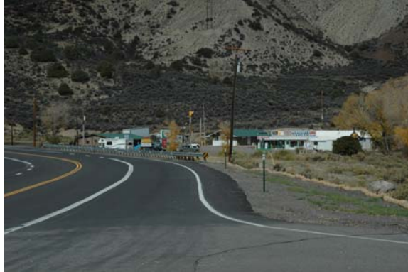
Figure 42. Off-site development, Post office and general store
