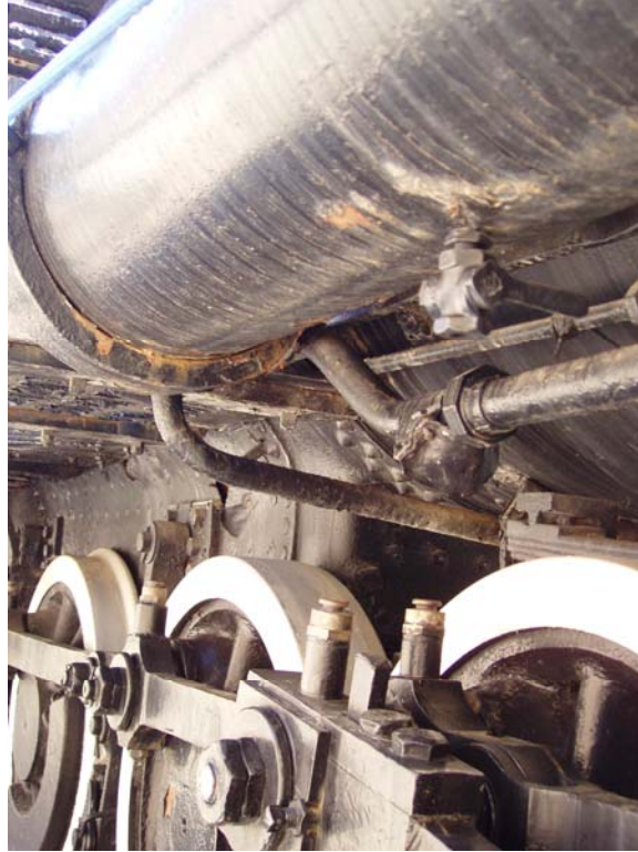
Figure 80. Rust under smoke box
