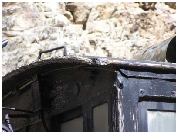
Figure 77. Weathered roof of engineer cab
