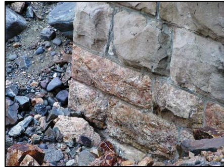
Figure 24: remnants of old granite pier
