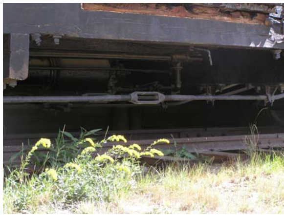
Figure 113. Truss rod and break cylinder
